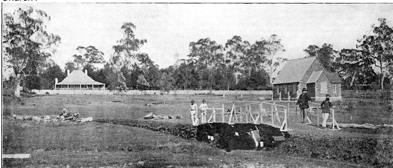
First Bridge across Rocky Pond Ck connecting town and Church of England 3
