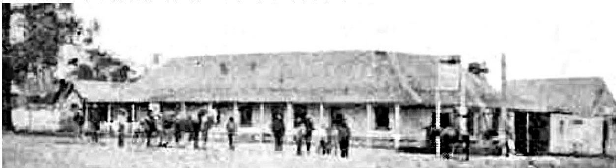
Old Telegraph Hotel Glen Innes. Original replaced by Grand Central c1875.
